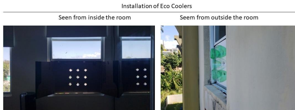
Fig. 5. Installation of the Eco Coolers seen from inside and outside of the room.
